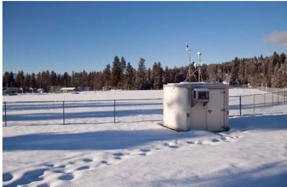
Photo of BAM at Seeley Lake Elementary School Site
